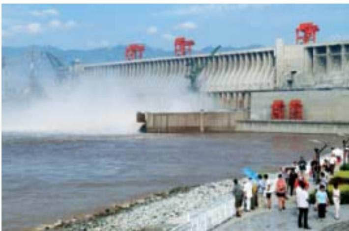
When too much water builds up behind the dam, the **spillway** allows the excess to flow around or through it and prevents the dam from breaking.
